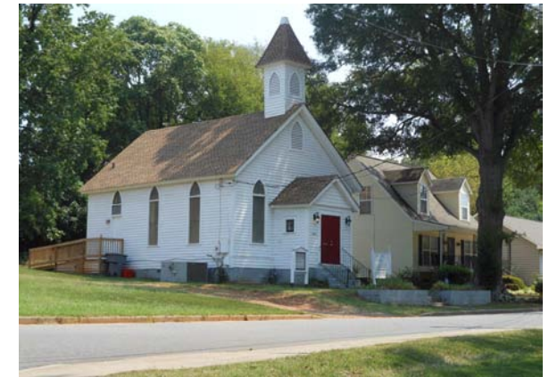
The Mount Zion Lutheran Church building is a local landmark in adaptive reuse as an office.
