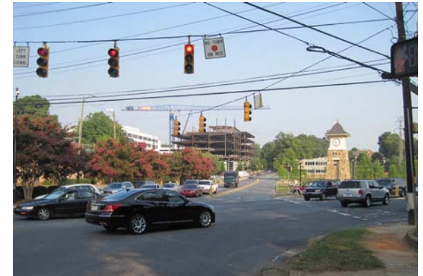
The Kings Drive/East Morehead intersection needs additional enhancements for safety and operation.
