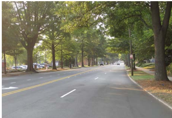
Trees and sidewalks back from the curb on East Morehead are ideal, but there is no room for bike lanes.
