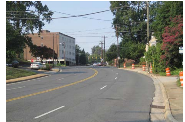
Construction barrels follow the edge of this street to be widened by a City bond project. The project will slightly widen the street to add bicycle lanes, plus left turn lanes at the new Pearl Park Way intersection.
