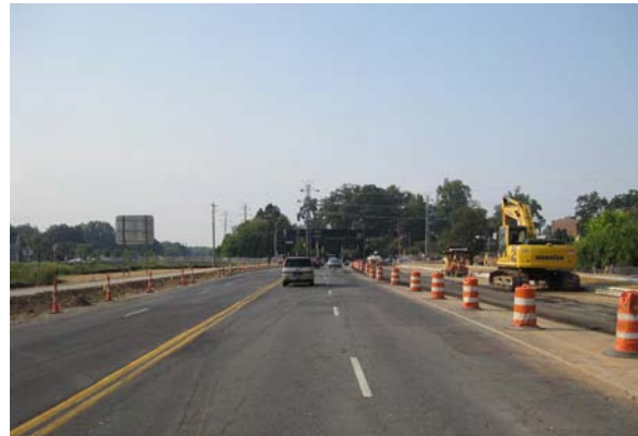
Bicycle lanes under construction on Kenilworth Avenue need to be extended into a few remaining blocks.
