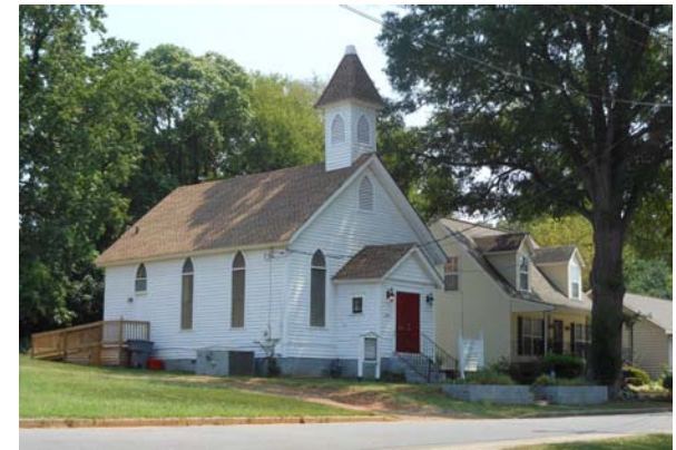
A historic church has been revitalized and enjoys new life as an office space in the neighborhood.
