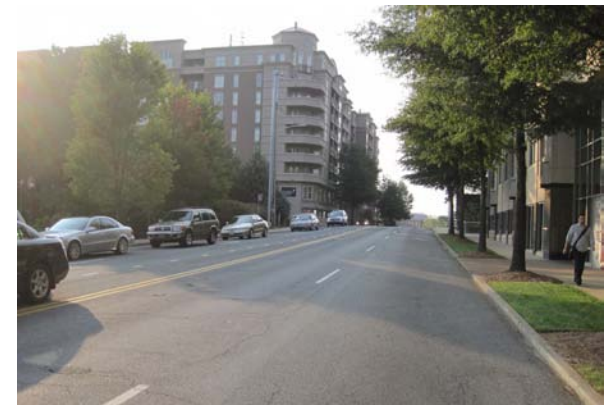
This section of East Morehead Street has multi-story buildings fairly close to the street, sited at the back of sidewalk and planting strip.
