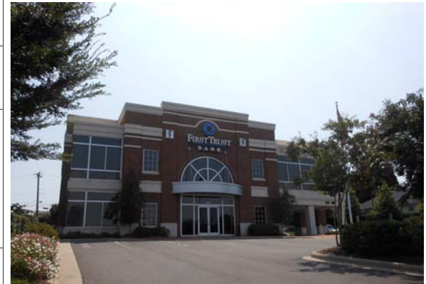
A freestanding bank that addresses the street and has a drive-thru in the rear makes for ped-friendliness
