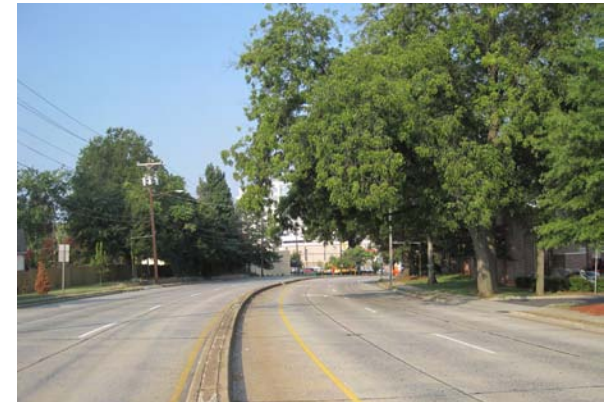
Formerly Independence Boulevard, parts of Charlottetowne Avenue still have visible remnants of Charlotte's oldest urban expressway. Remnants along this section include a wide concrete road bed and a raised traffic median.
