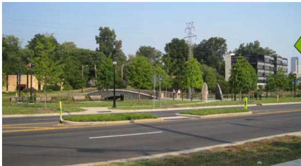
A pedestrian refuge island at Kings Drive and Baldwin Avenue is a model for additional crossings.
