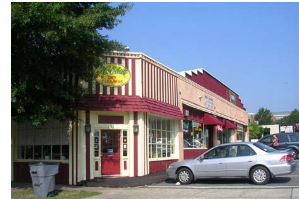
Older strip retail along East Morehead Street has little in the way of landscaping along the front.
