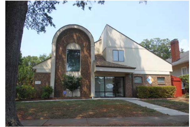
A contemporary infill office development in the Cherry neighborhood.
